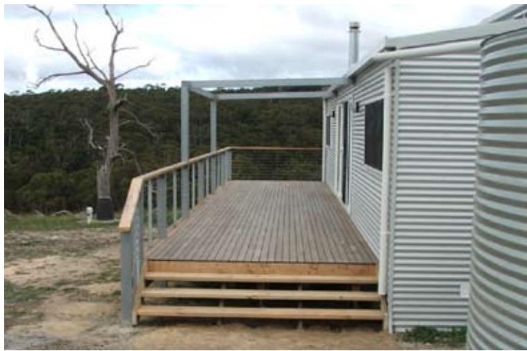
Photo: Sugar Gum decking in situ at Deans Marsh, Victoria
